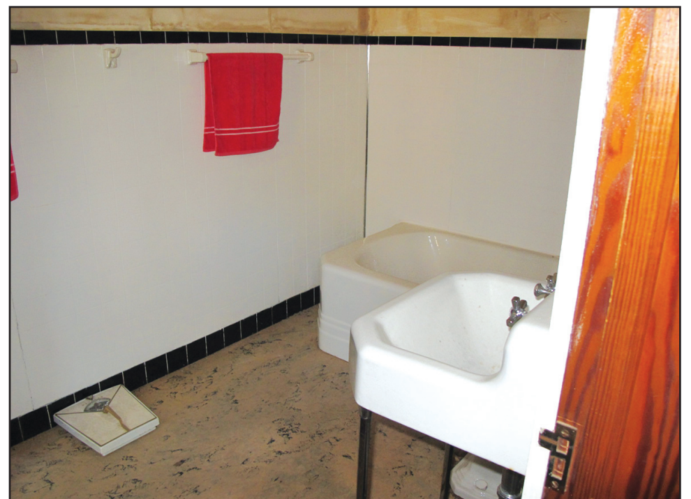
The downstairs bathroom before
